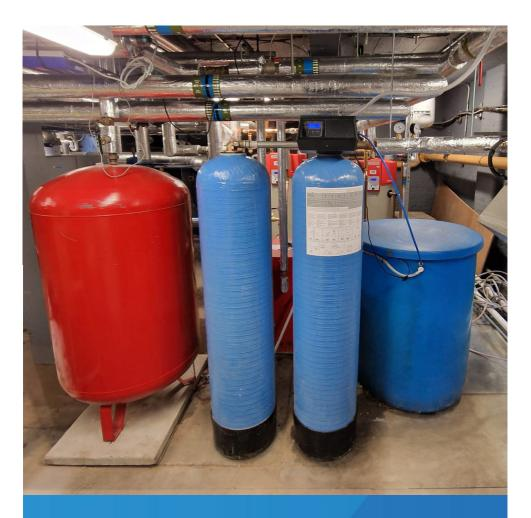
Installed borehole filtration that included 5 Micron filters, Carbon media and an Ultraviolet system. Laboratory analysis has proved the effectiveness of the install and water quality is up to the required standard to supply the hospital.
